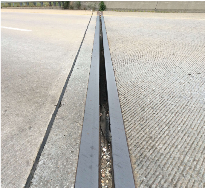
PHOTO 1 Description Compression joint seals have failed at the East and West abutments. They leak water and dirt on the abutments.
