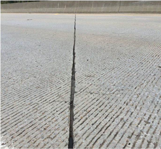
PHOTO 1 Description The deck saw joints are deteriorating and leak water that appears to be causing active corrosion in the metal stay in place forms.
