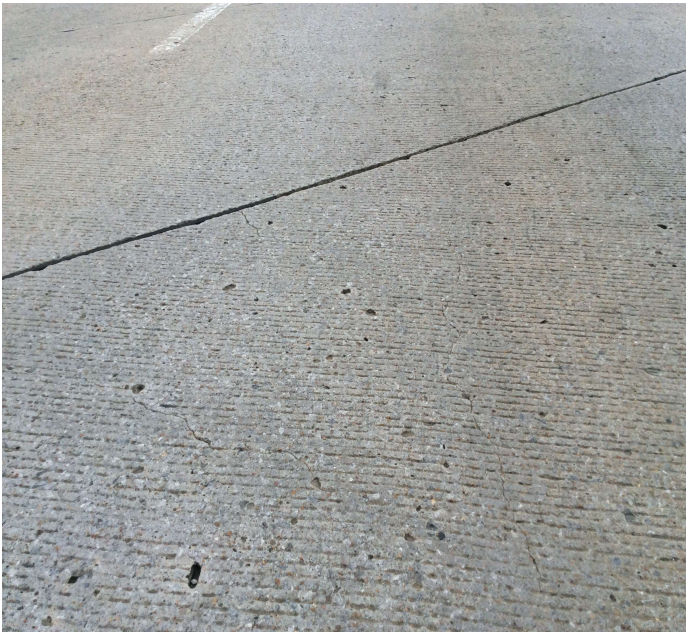
PHOTO 1 Description Deck has sealable cracking.
